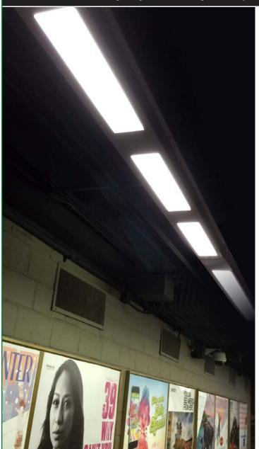
There are three components to the METRO Platform Light: LED Module, Fixture Frame and Raceway.
