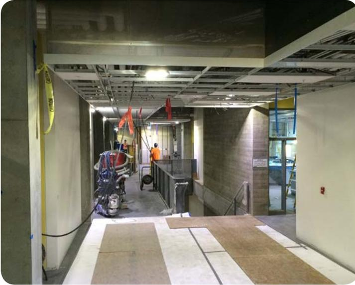
The electrical contractor buried the power cable in the slab and ordered the lighting fixtures with 10' whips. This combination simplified the initial installation and on-going reconfiguration of the lighting fixtures.
